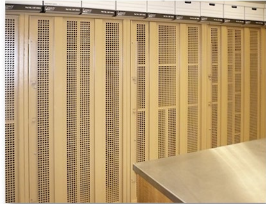
EXAMPLE 11F: Pass-through Temporary Storage Lockers (Rear view)
